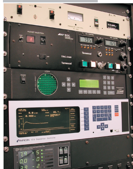
Control panel of a Meade UHTC electron-beam vacuum coater.
