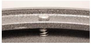
Figure 18. The primary mirror collimation screws are the ones with the springs visible just under the mirror cell casting.
